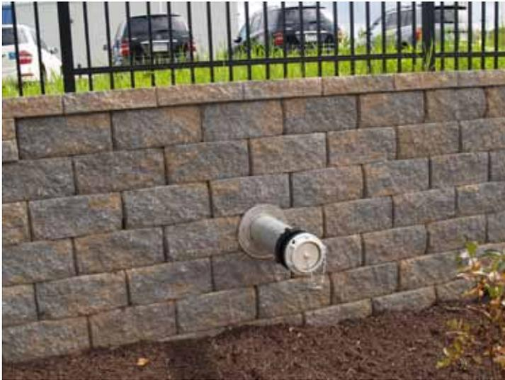
**A dry fire line was installed 80 feet into the retaining wall.**
