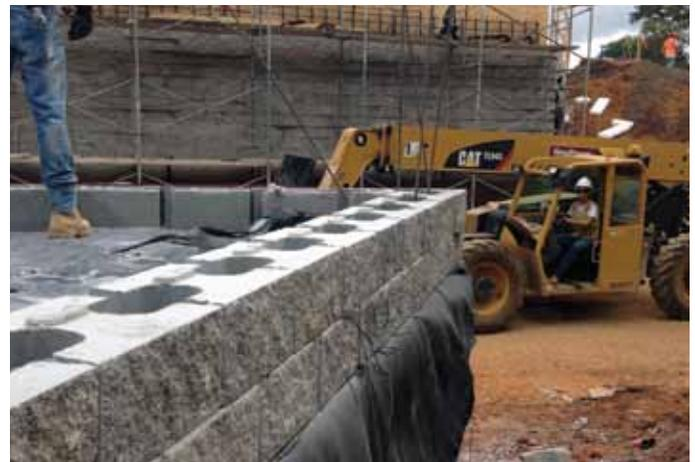
Special cuts in the Vertica® wall blocks were reinforced with rebar for the acute abutment walls.
