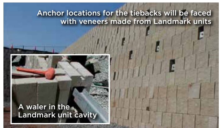
Installation of the tiebacks
