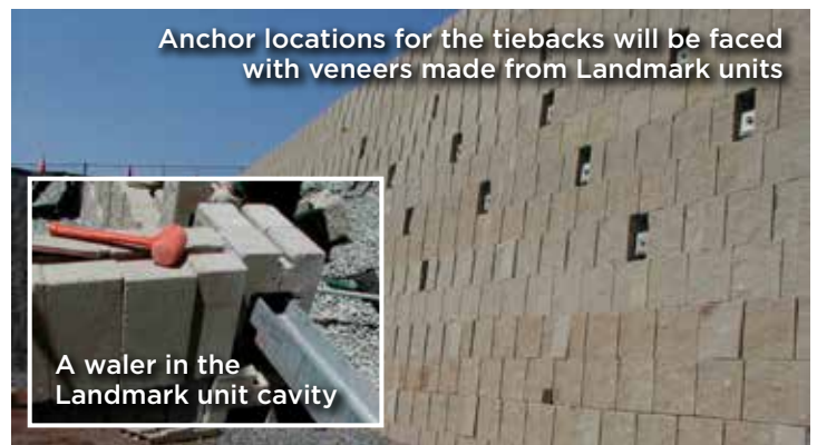
Installation of the tiebacks
