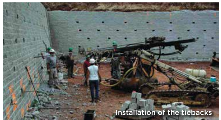
Anchor locations for the tiebacks will be faced with veneers made from Landmark units
