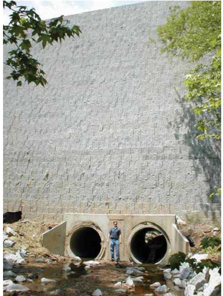
To provide drainage, this land bridge structure has two 6-foot-diameter culverts through the 61-foot-high walls.
