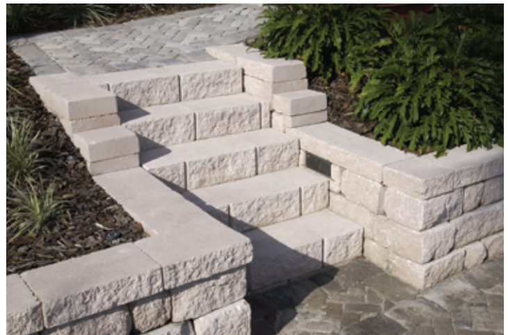
Light units were installed for safety on steps constructed with the Highland Stone® retaining wall system.
