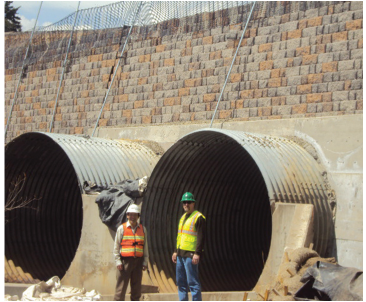
The challenging installation of this 65,000-square foot retaining wall occurred at the bottom of a slope and above a creek.
