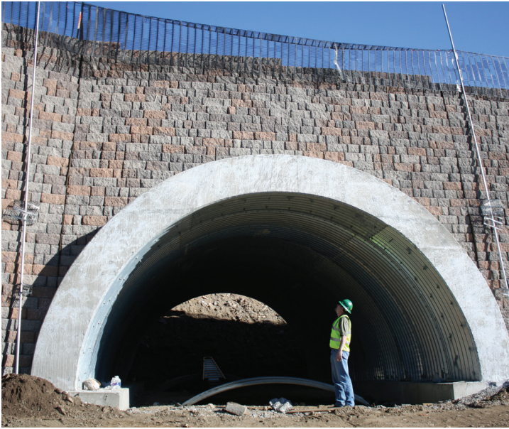
The retaining wall was built to accommodate large culverts for spring flooding and to provide a passage for wildlife.
