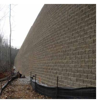
One of the first walls built was a 48-foot-tall (30,000 sq. ft.) Diamond Pro Stone Cut® retaining wall.
