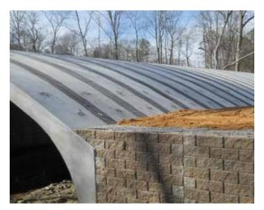
Bridges were constructed with massive, 50-foot-wide arch culverts and the Vertica Stone Cut retaining wall system.
