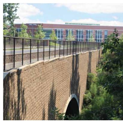
The Vertica Stone Cut<sup>®</sup> retaining wall system integrates with arch culverts to preserve wetlands and support three road bridges.
