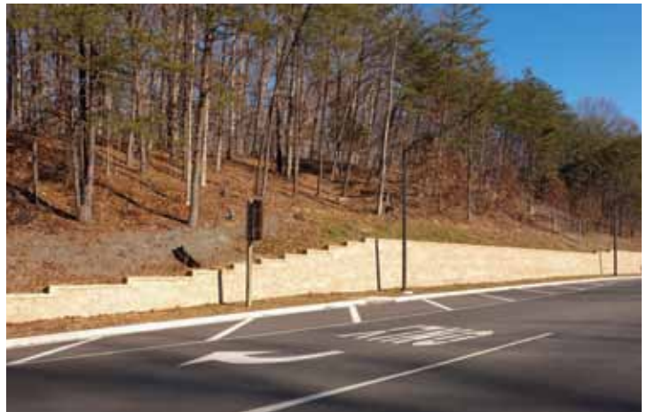
The finished wall is an important and attractive component in the widened road.
