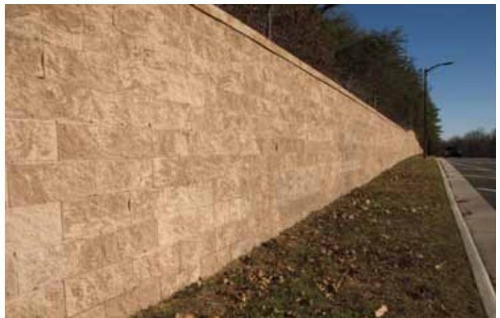
The Anchorplex retaining wall system built with Vertica® products made it possible for the road to remain open during most of the construction.
