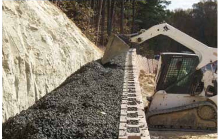
The Anchorplex™ retaining wall system can be used to build in areas too small for extensive excavation.
