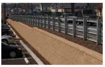
Using the Anchorplex retaining wall system with Vertica<sup>®</sup> products created a vertical structure with room behind for the required sidewalk and handrail along the state road.
