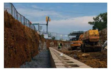
Using the Anchorplex<sup>™</sup> system made it possible to build this wall next to a state highway without extending reinforcement into the right-of-way.
