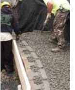
The structural backfill was poured in lifts behind the wall and into open areas in the blocks.
