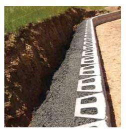
The Anchorplex™ system is a unique retaining wall system built with Anchor™ products and structural backfill that extends the depth and mass of the retaining wall.
