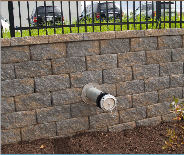
A dry fire line was installed 80 feet into the retaining wall.
