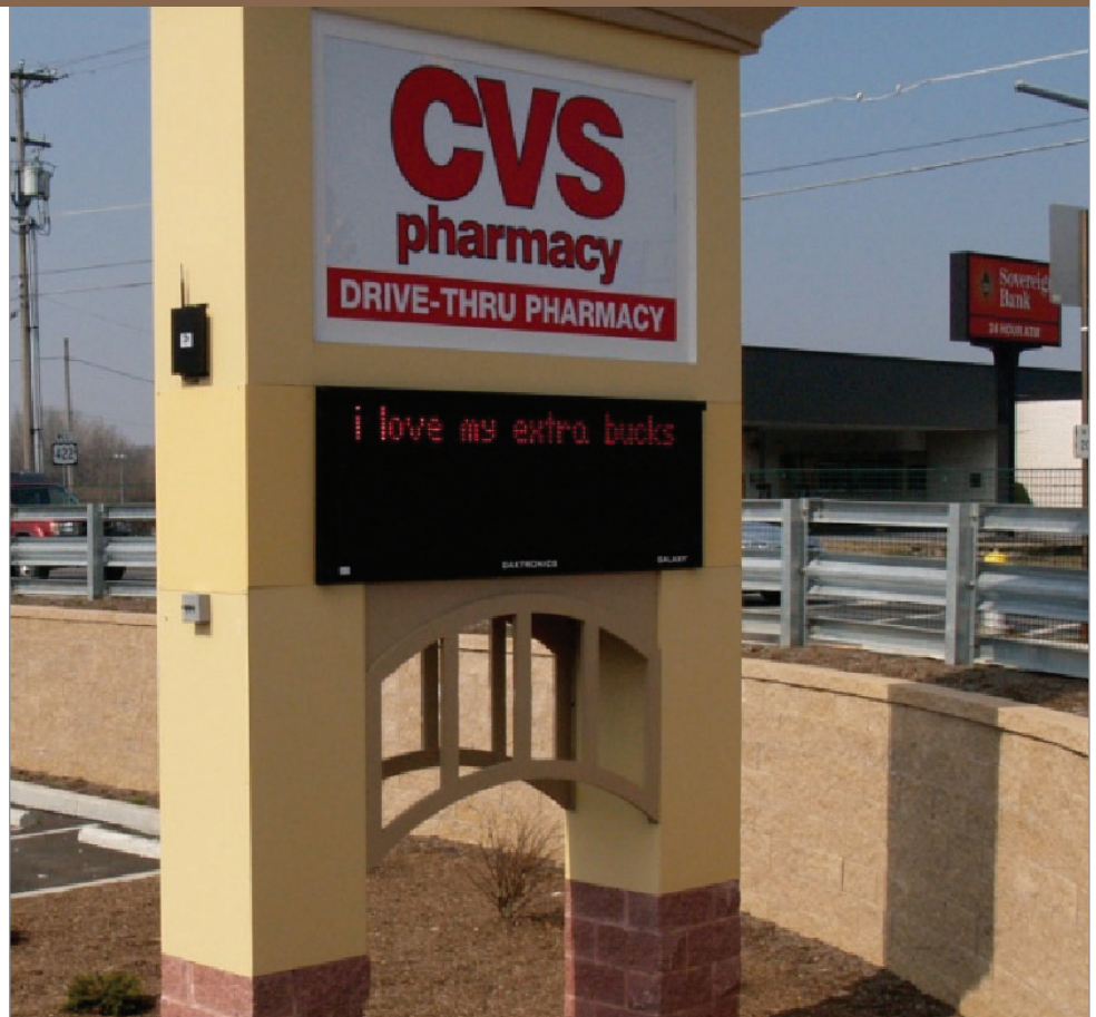
This Anchorplex™ retaining wall system next to a busy state highway was constructed with Vertica® wall units.
