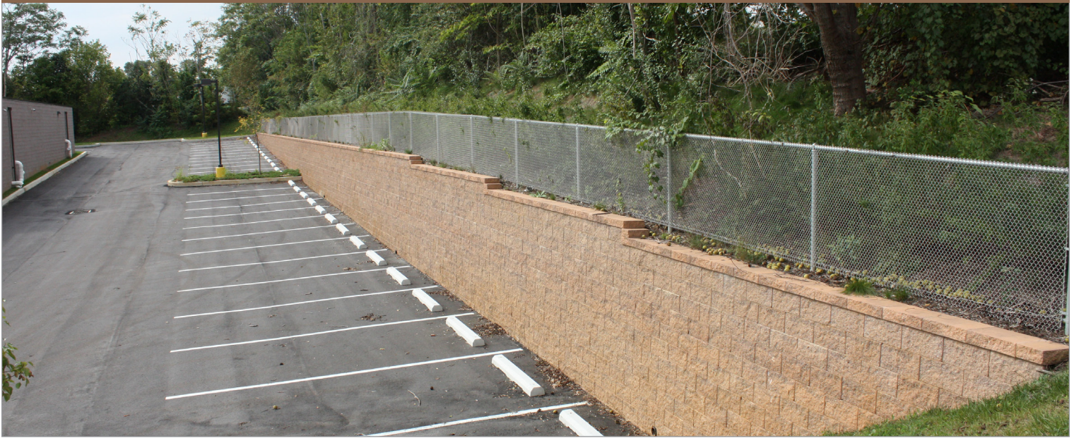
A traditional segmental retaining wall requires significant excavation, but the Anchorplex™ retaining wall system uses structural backfill and requires less excavation.
