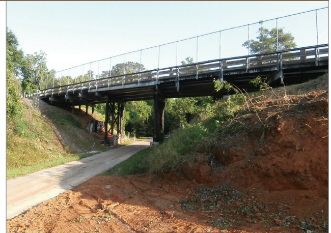
Before image of the Orange Avenue bridge crossing and site limitations.
