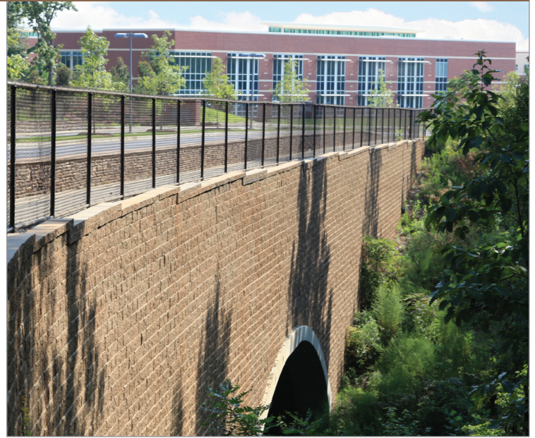
The Vertica Stone Cut® retaining wall system integrates with arch culverts to preserve wetlands and support three road bridges.
