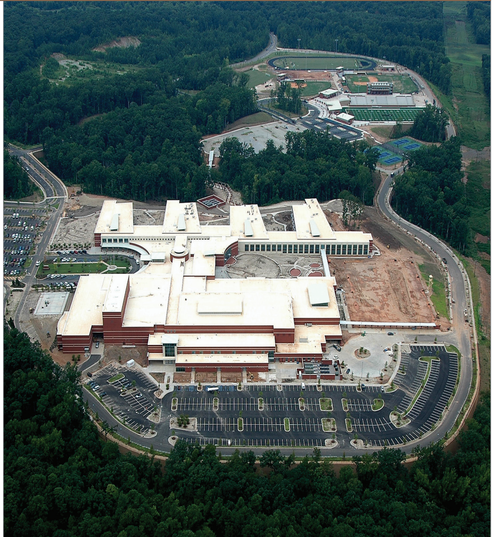
More than 100,000 square feet of Diamond Pro Stone Cut® retaining walls circle the River Bluff high school campus.
