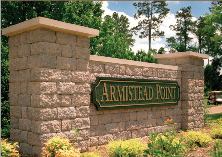
The blended, earth tone colors and unique, rustic appearance let to other applications on the project such as pillars and the entrance sign on the property.
