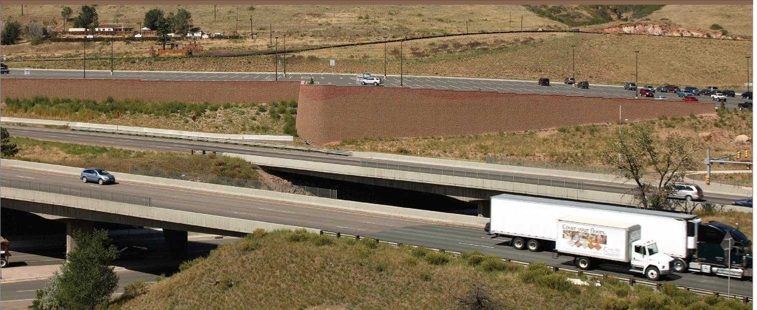
The design used a multipiece system to mimic area rock outcroppings. Four custom colors were used in the wall to show a sweeping motion near the top, which blends seamlessly with the surrounding scenery.
